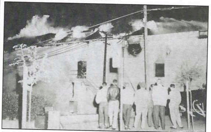
Fireman play their hoses on the doctor's offices, reducing the chances of spreading to the venerable Methodist Church next door. Mayor John Nelson turns out to be a fire buff (see if you can spot him), as flames leap through the roof of the theater. Photo by Wm.Morgan
