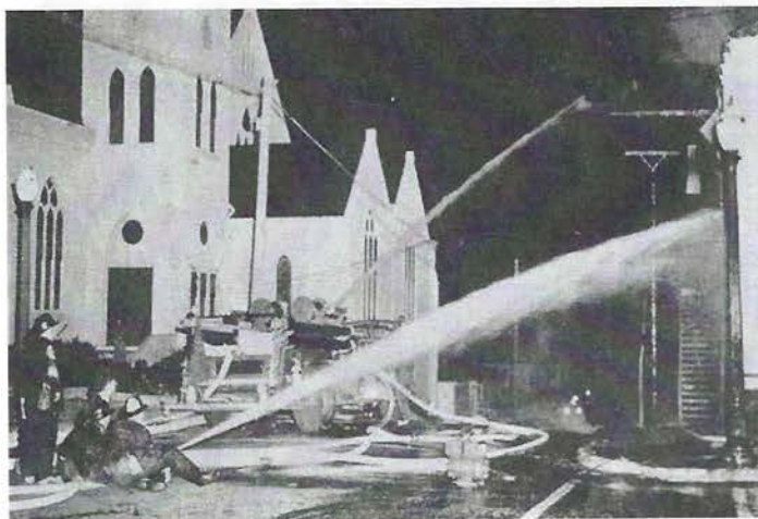
Fireman Al Page '29 and Harold Compton '35 arch water into the building, where it still smolders. Photo by: Don Stevens
