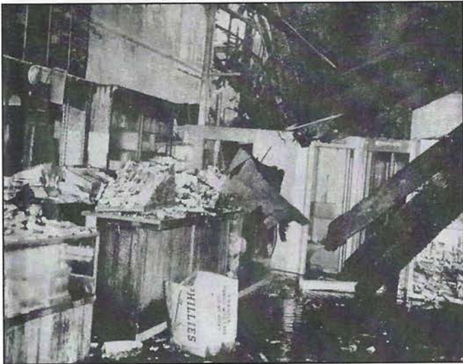
Interior of John Stewart's shop, completely ruined by the fire. Photo by: Don Stevens
