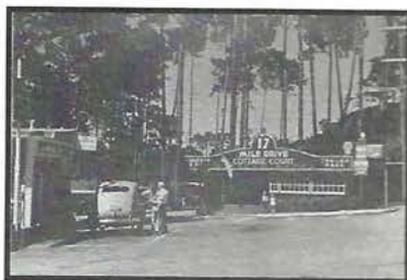
Gas Station on left.
