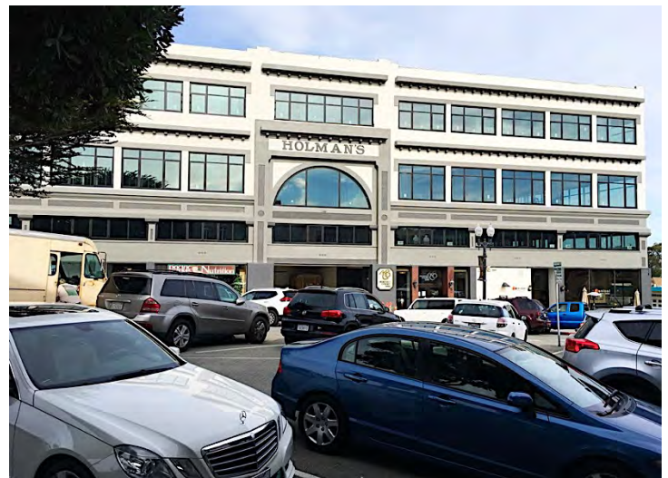
The windows have been completed in the Holman Building since our last issue! The architects have been successful in restoring the building to its 1940s appearance. Photo by Joanie Hylar '68. More at www.theholman.com .
